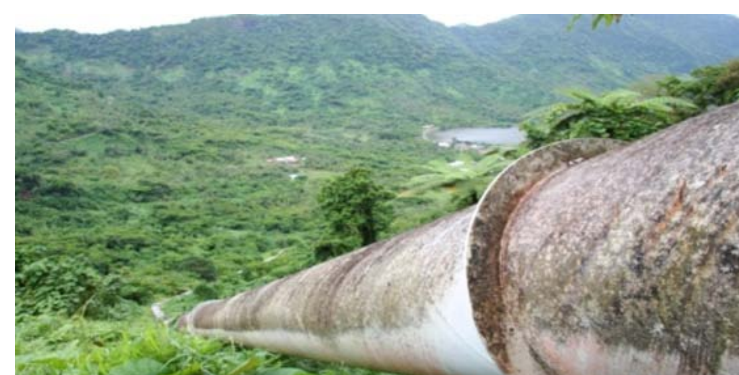
Penstock connecting Afulilo Dam to Taelafaga Powerhouse, Yahya Abawi.
